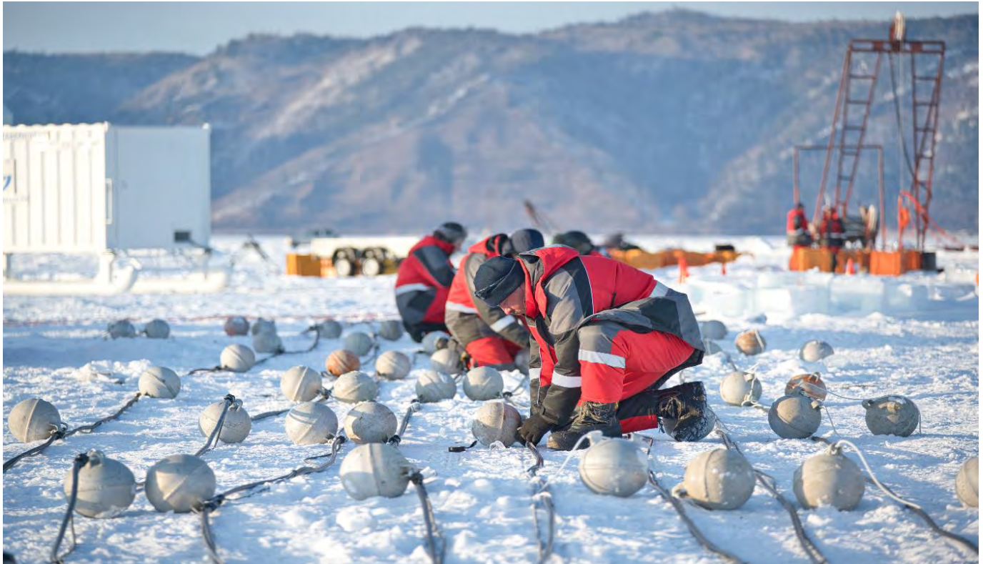
Fig. 12. Assembling the Baikal-GVD installation cluster garland
