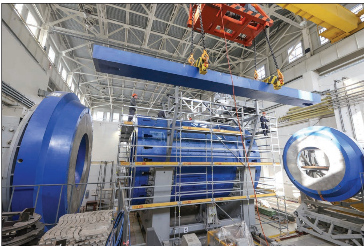
The Veksler and Baldin Laboratory of High Energy Physics. Installation of the last three beams of the magnetic core of the MPD detector
